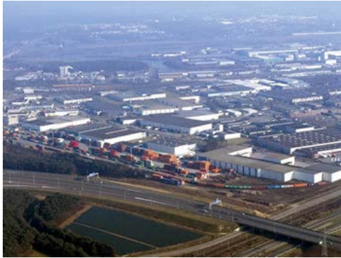
Venlo Intermodal Terminal
