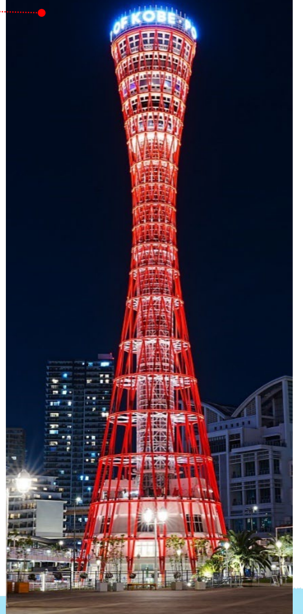
(4) Renovated Kobe Port Tower
